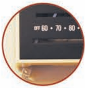
Lowering your thermostat by one degree in winter can save around 6% of heating energy usage.
