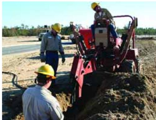
**Underground Lines** - Numerous requests for underground service came in 2008 from builders of new apartment complexes and neighborhoods in west Jackson County. Underground lines are aesthetically pleasing since they are not seen, but these lines cost more than overhead lines because of the insulation needed to protect the wire and make it more durable in the ground. Underground lines also take more time to install.
