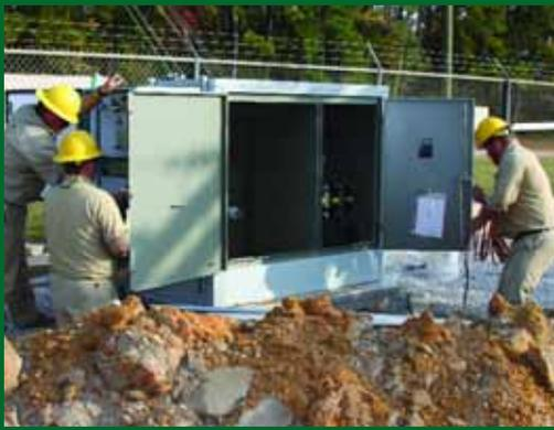
**AMR Hardware** - All new and upgraded substations are equipped with Automated Meter Reading (AMR) hardware, a necessary component of communicating electricity use readings from a member's meter to Singing River Electric's main office where billing takes place. In 2008, Basin, Big Point, Escatawpa South, Forts Lake, Helena, Hickory Hills, Kittrell, Lucedale South, Monaco Lake, Orchard Road, Rocky Creek, Sand Hill, Sawmill, State Line and Wade substations had AMR hardware installed.
