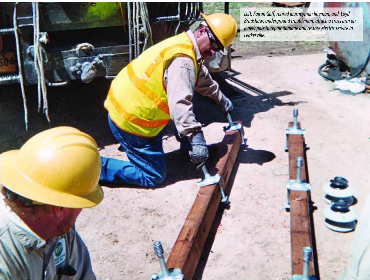
*Left: Fairon Goff, retired journeyman lineman, and Loyd Bradshaw, underground troubleman, attach a cross arm on a new pole to repair damage and restore electric service in Leakesville.*
