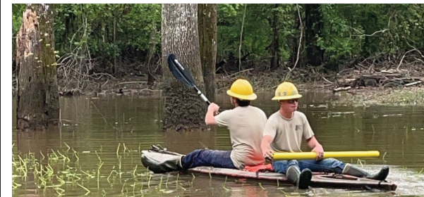
Linemen Colby Pilkington and Collin Davis join Construction Foreman Ryan Evans to restore power in Cedar Creek Estates in Jackson County.
