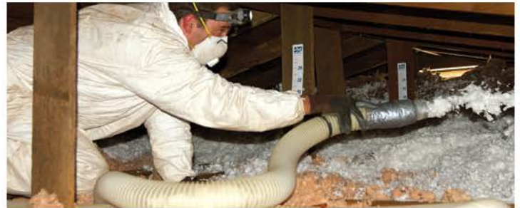
Prioritize the invisible upgrades that make your home more comfortable and efficient, such as adding blown-in insulation to your attic. Photo: Bonneville Power Administration
