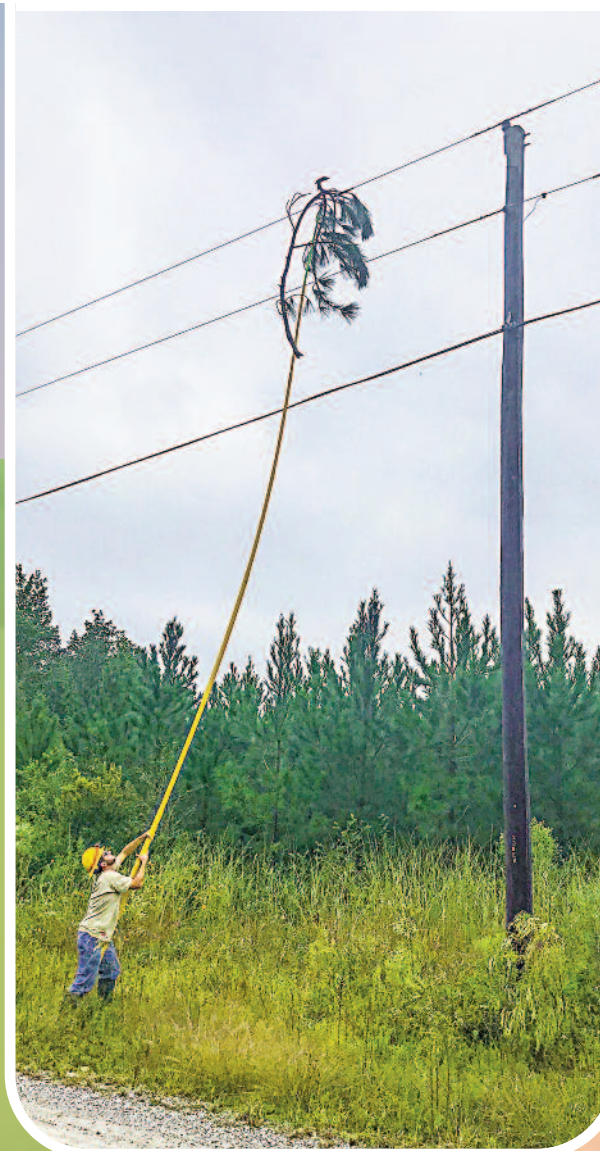
Serviceman Ryan Bounds removes a limb from a power line in the Shipman community in George County.
